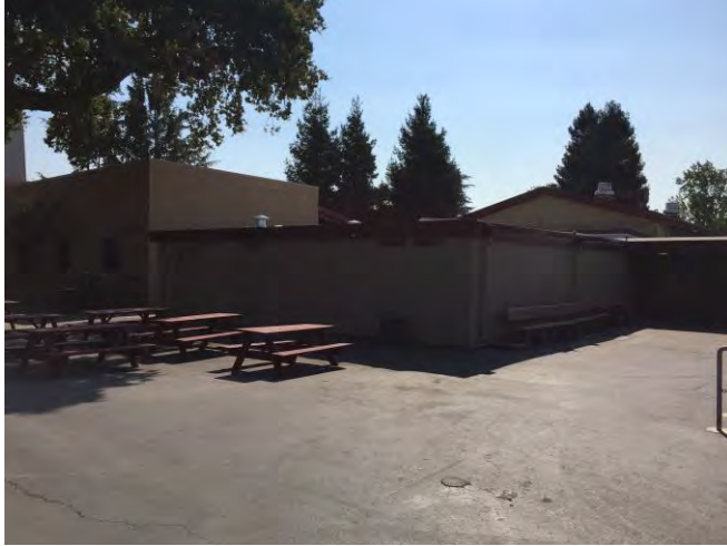
Photograph 11. (looking southwest). Bathroom building.
