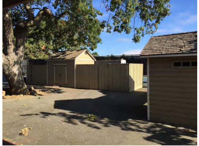
Photograph 2 (looking northwest). Sheds south of tennis court in Area 1. Top of emergency generator can be seen behind wood fenced enclosure.
